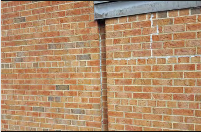
Photo No. 1: HAN600 – Grey Caulk, at Expansion Joints
