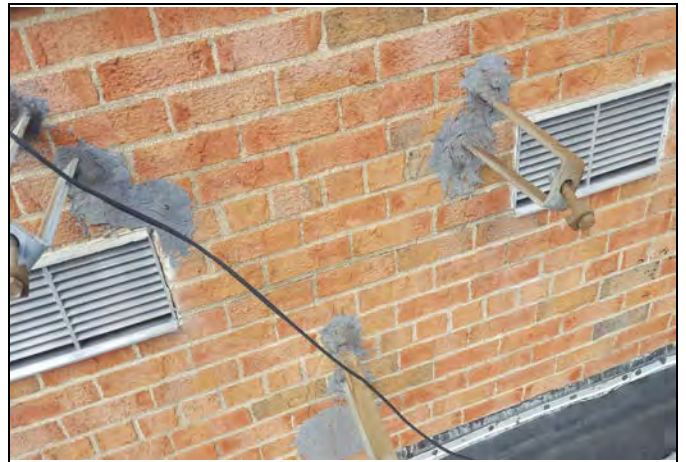
Photo No. 4: HAN710 – Roofing Cement, at Hanger Penetrations
