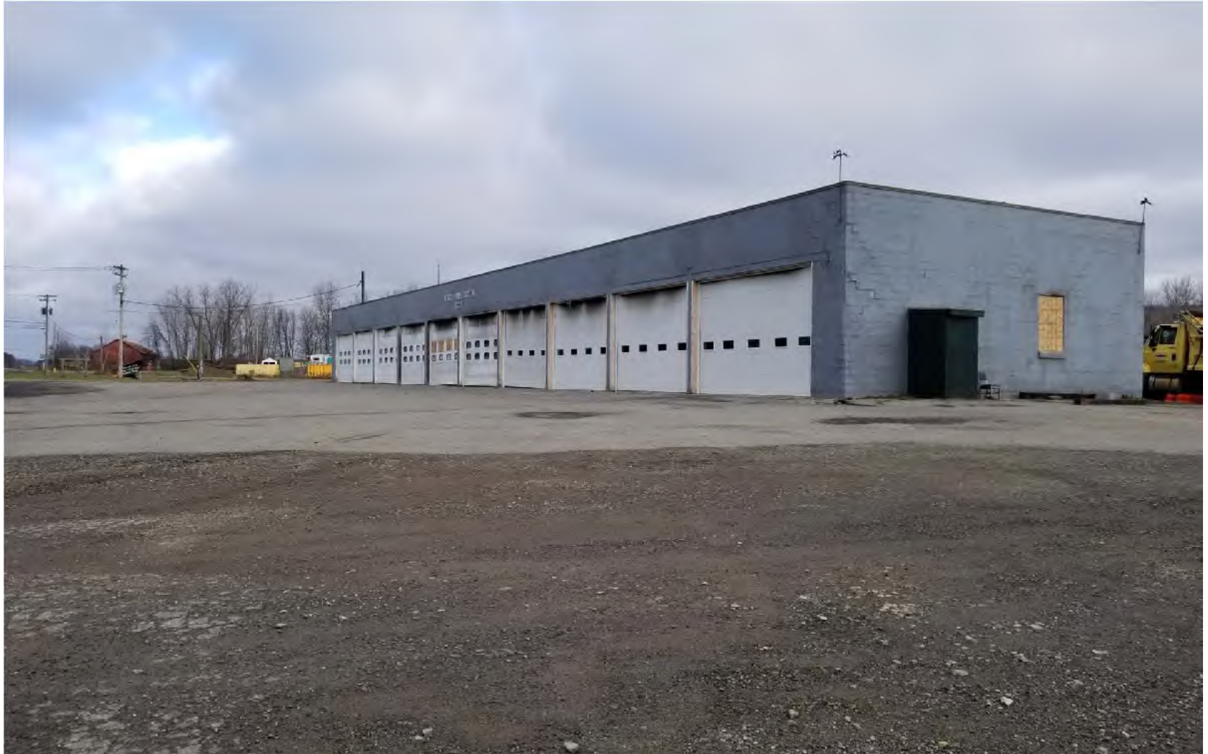
8600 NYS Route 16 Highway Barn, South West Corner
