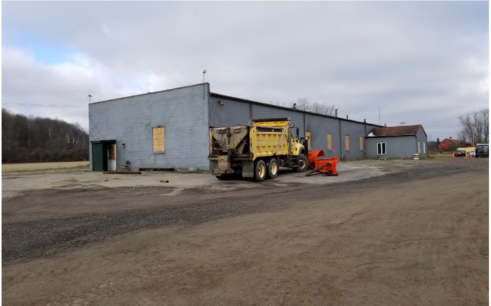
8600 NYS Route 16 Highway Barn, South East Corner
