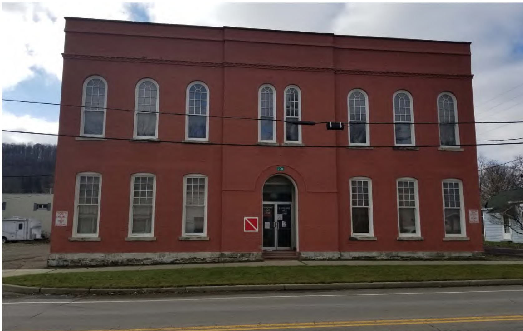
200 Erie Street, Front Facing Erie Street, North East Face
