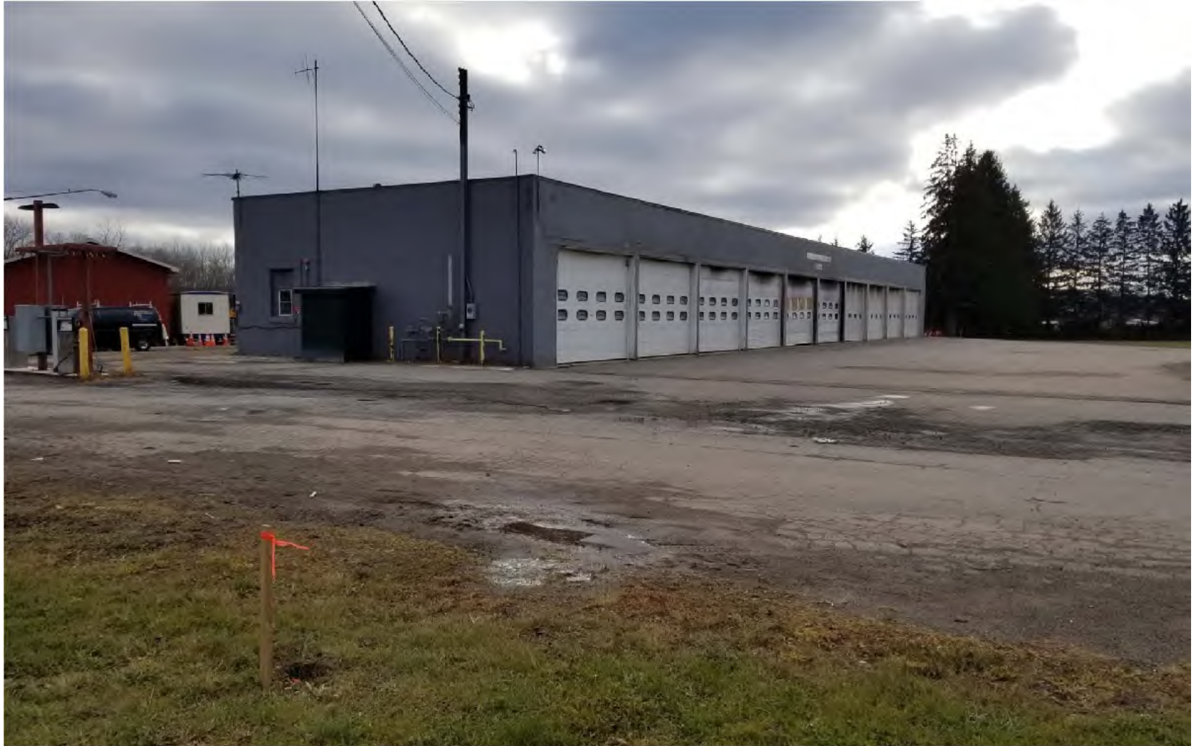
8600 NYS Route 16 Highway Barn, North West Corner
