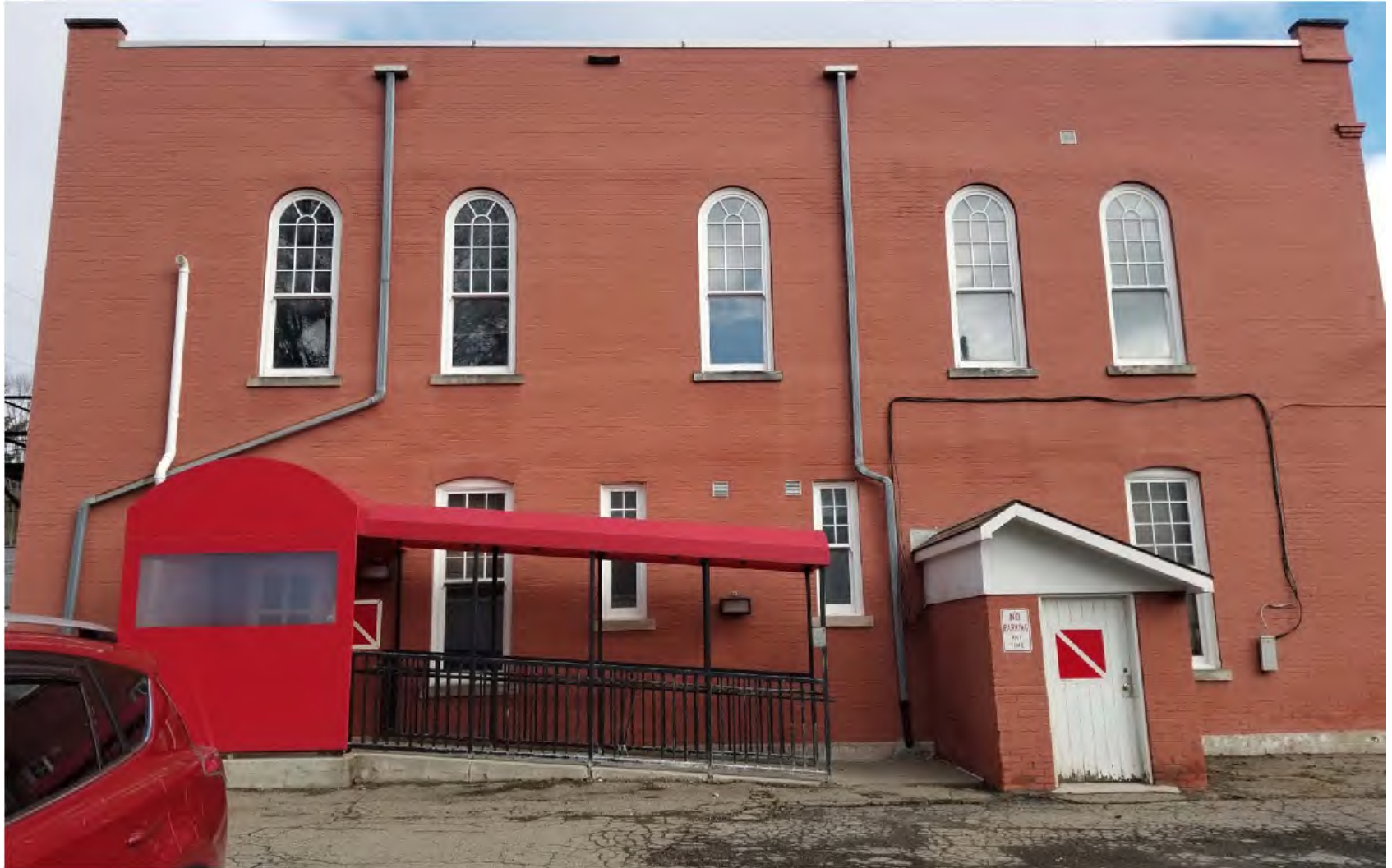
200 Erie Street, Rear Entrance, South West Face
