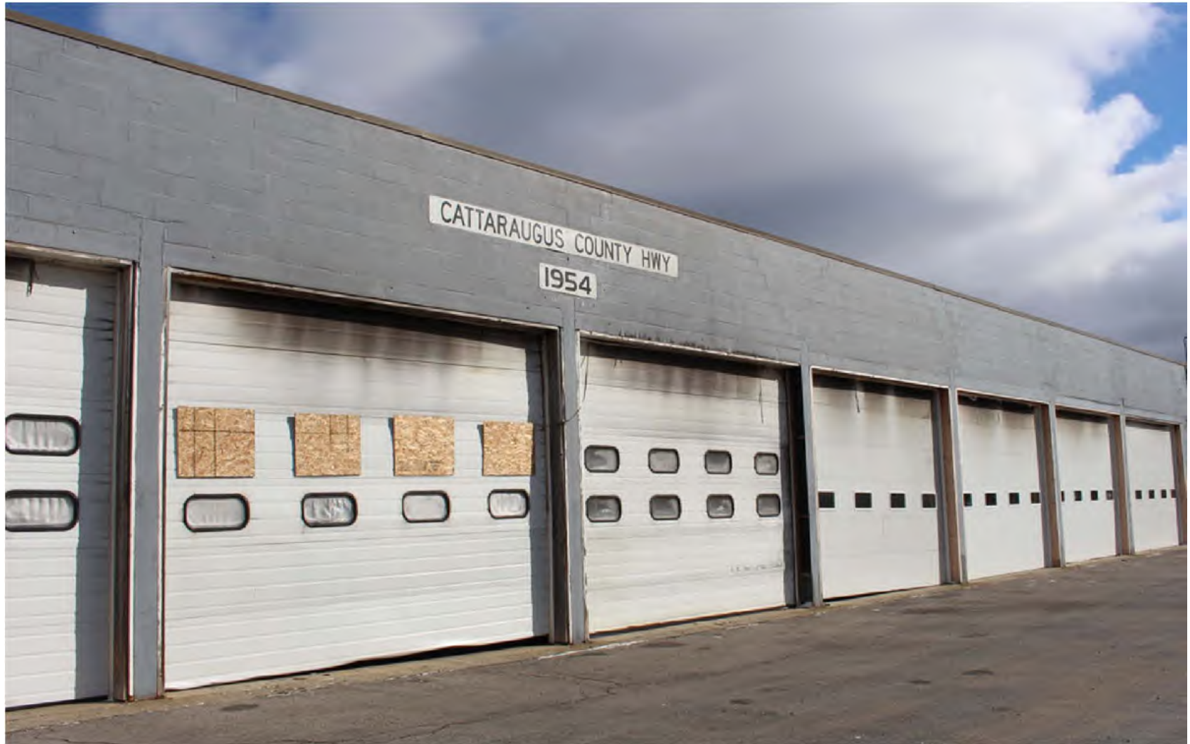
8600 NYS Route 16 Highway Barn, Front facing Route 16, West Side
