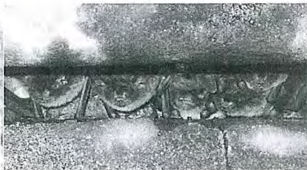
Photo 2: Visible bats within an expansion joint
