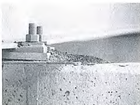
Photo 5: Guano deposit on pier, obscuring structural features.
