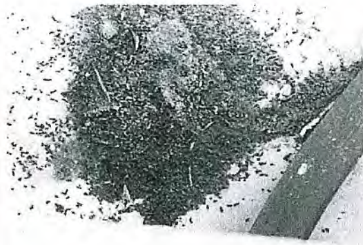
Photo 4: Guano deposits visible from bridge deck, on top of pier
